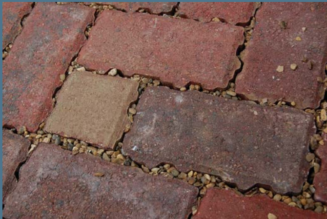
Permeable driveway surface.
